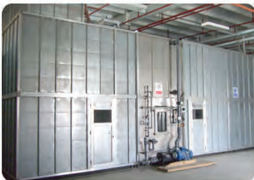
The largest air handling unit 16 m Long x 6.6 m Wide x 4.5 m Height
