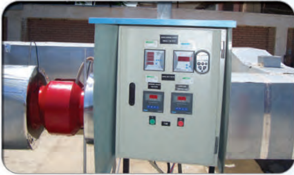
Test Station for Smoke Fans
